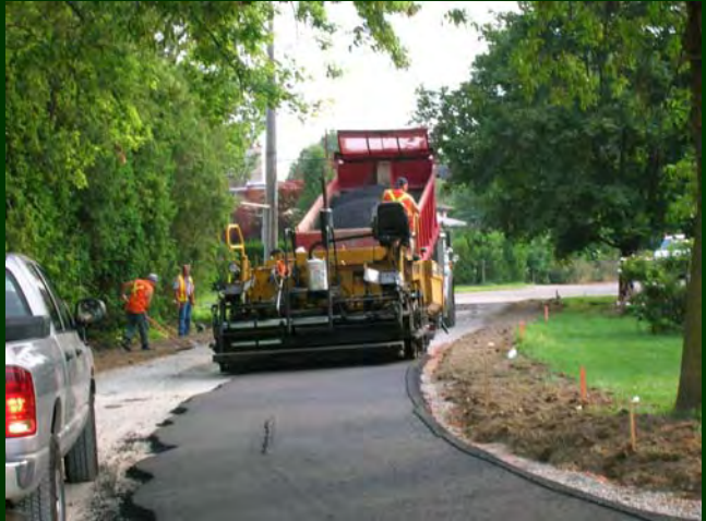
DELIVERING THE ASPHALT ON A HOT SUMMER'S DAY.
